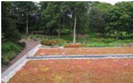
Extensively green roof—Botanic Gardens
