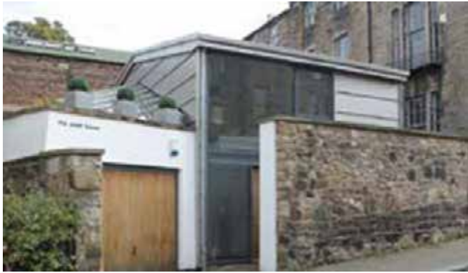
Incorporating a boundary wall—Hart Street
