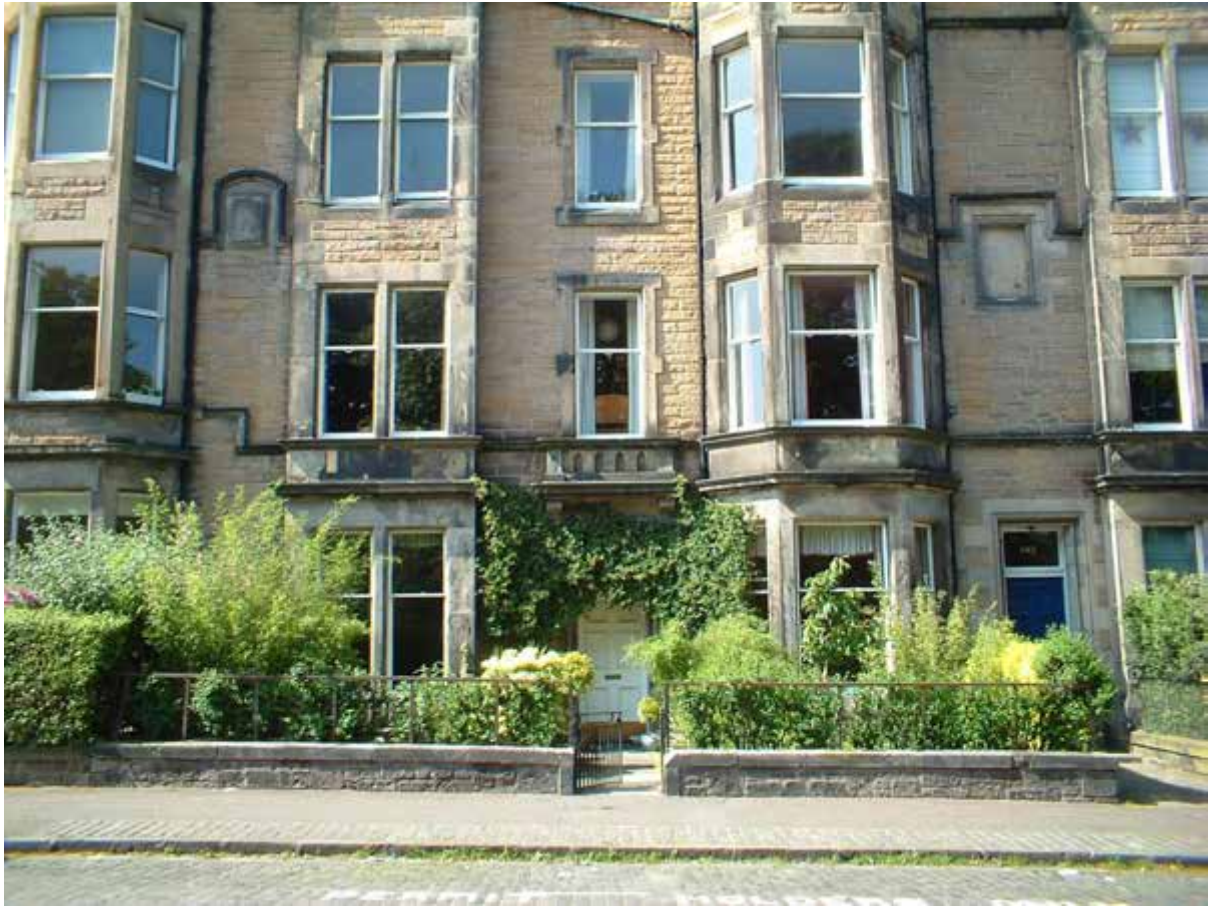
Active frontages and housing— Forbes Road Marchmont Tenement
